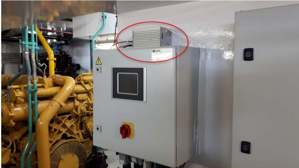
Figure 3. Smart Emissions Measurement System (SEMS). Small box on top of the engine control cabinet
